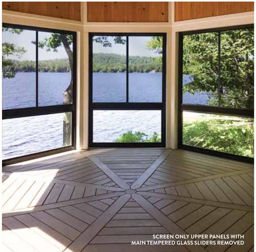
SCREEN ONLY UPPER PANELS WITH MAIN TEMPERED GLASS SLIDERS REMOVED
