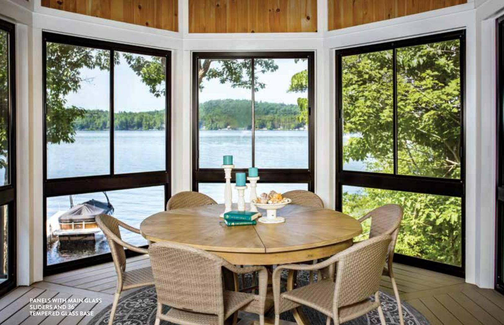
PANELS WITH MAIN GLASS SLIDERS AND 36" TEMPERED GLASS BASE
